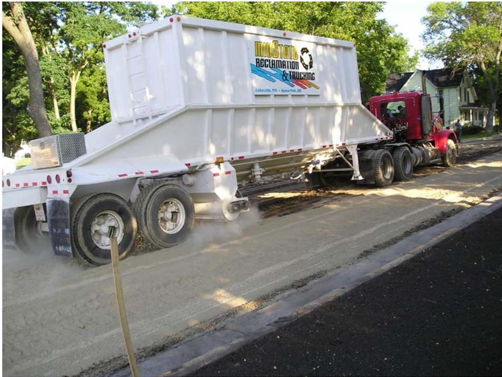
Fig. A1-2. Lay-down truck placing fly ash on RPM.
