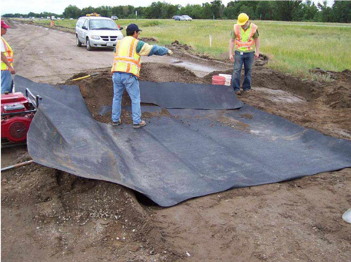
Fig. A2-3. Installing geomembrane for lysimeter.
