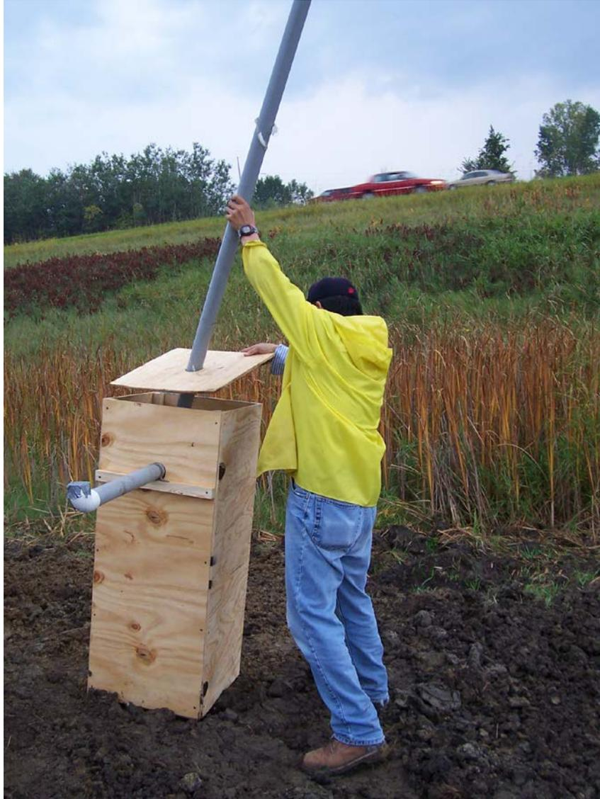
Fig. A2-6. Assembling leachate collection tank.
