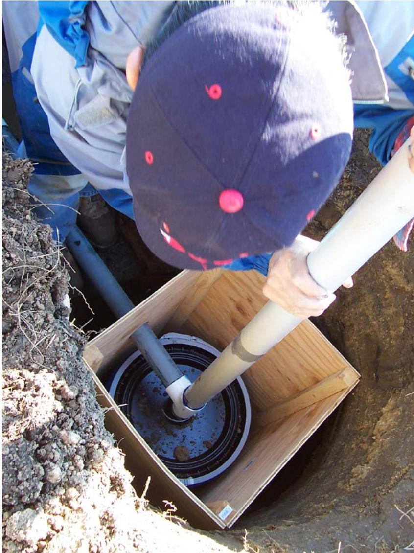
Fig. A2-7. Installing leachate collection tank.
