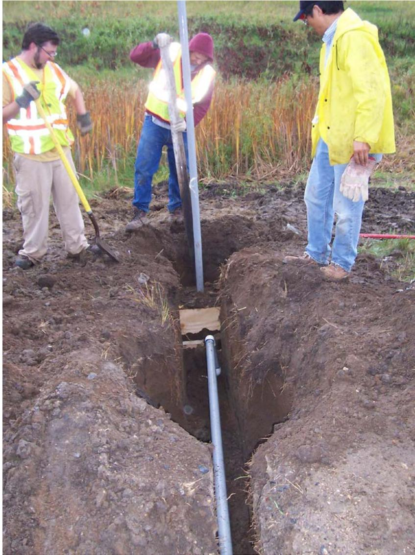
Fig. A2-8. Installing leachate collection tank.
