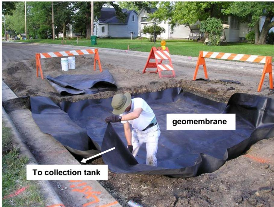
Fig. A1-7. Installing geomembrane for lysimeter.
