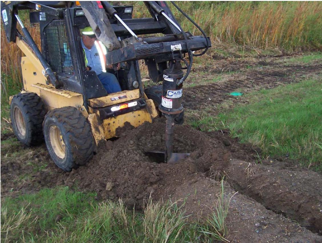
Fig. A2-5. Preparing hole for leachate collection tank and trench for drainage pipe.
