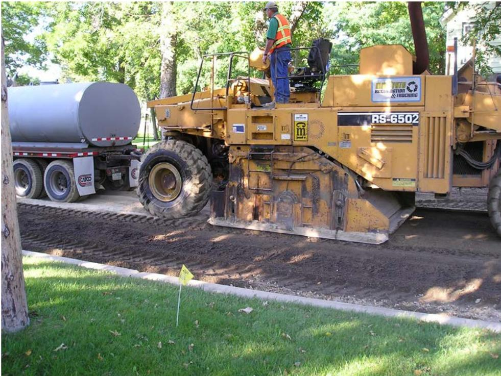
Fig. A1-3. Water truck and road-reclaimer blending fly ash, water, and RPM.
