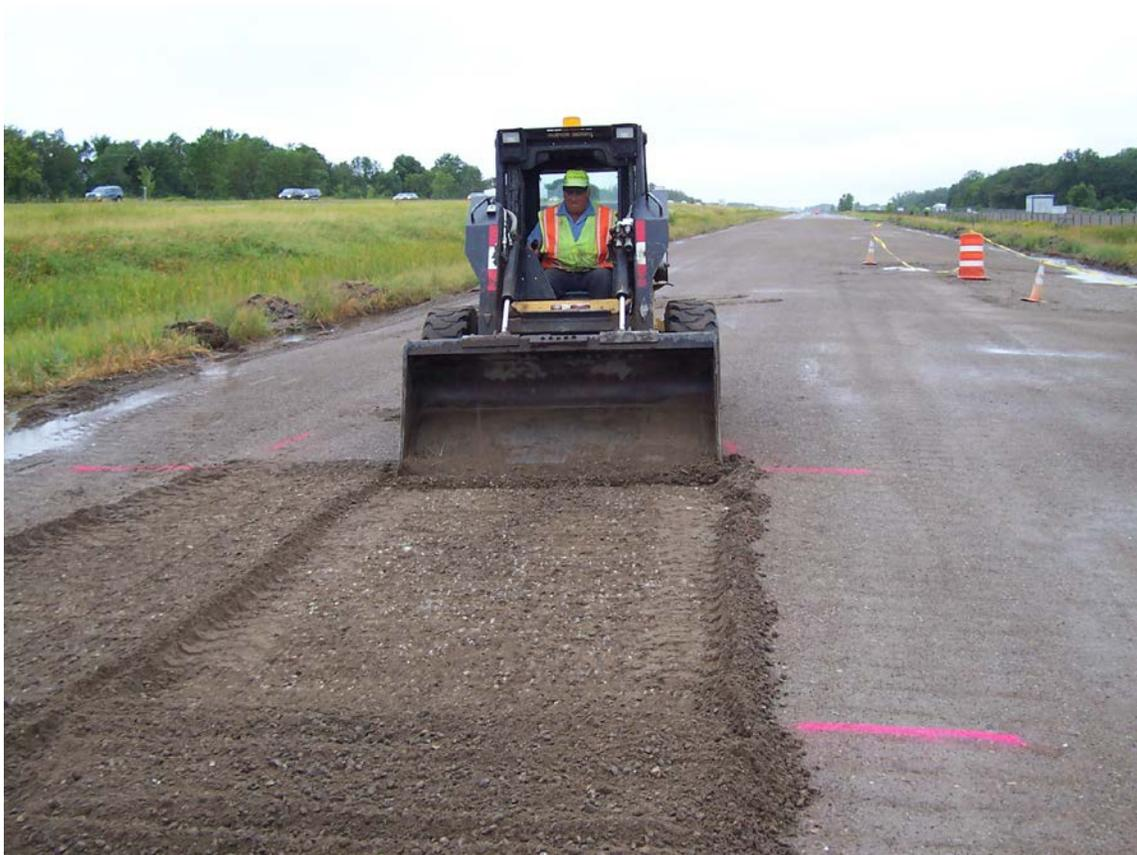
Fig. A2-1. Preparing indentation in sub-base for lysimeter geomembrane.
