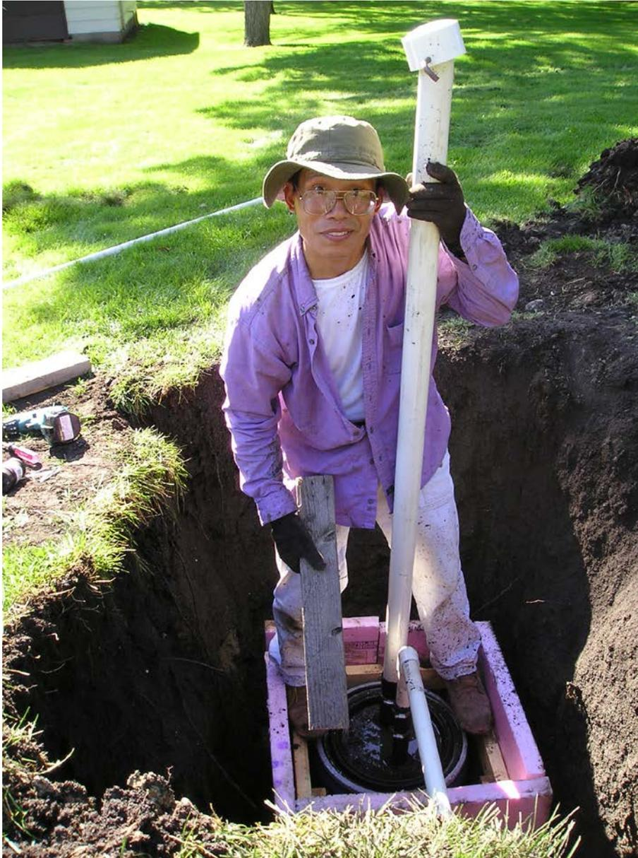
Fig. A1-8. Installing collection tank for lysimeter.
