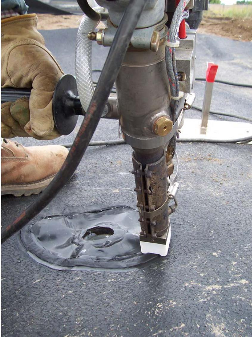
Fig. A2-4. Welding geomembrane to lysimeter drainage pipe assembly.
