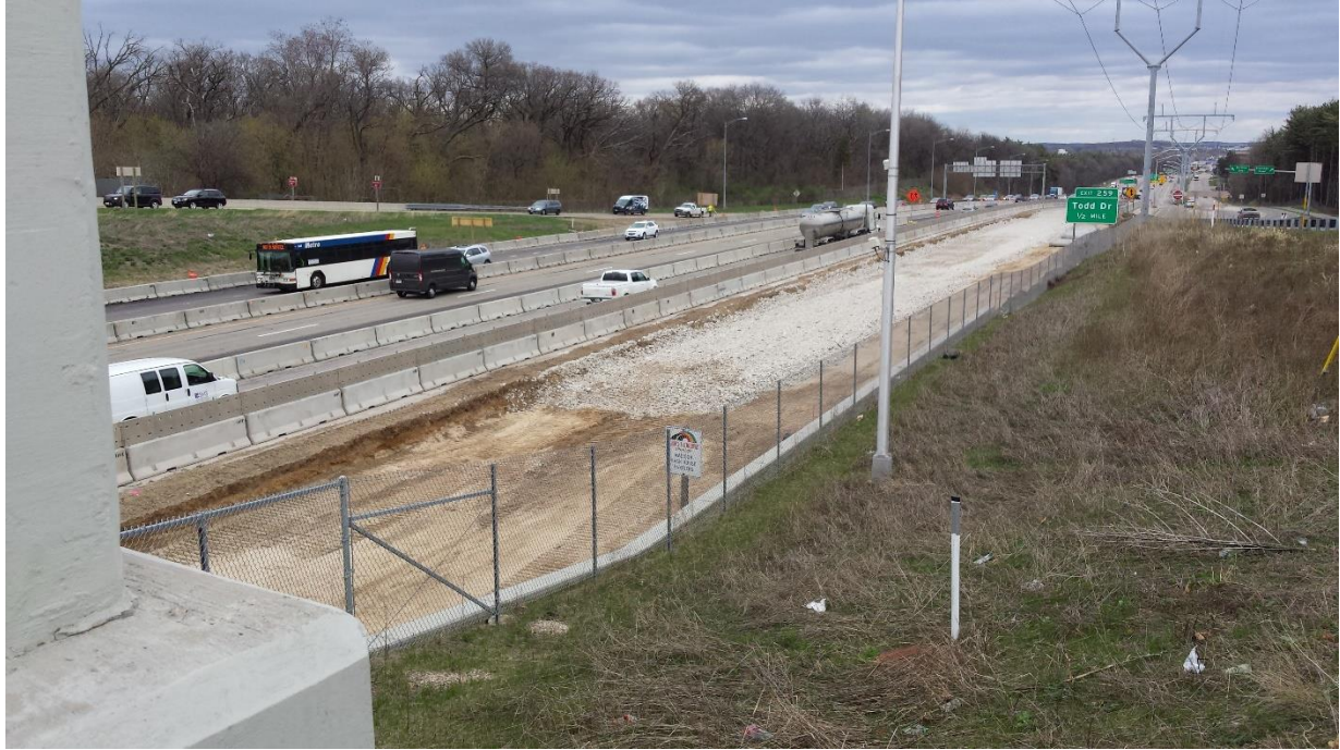
Figure C13. Aerial photo of eastbound Beltline reconstruction; base course is being placed (April 2015)
