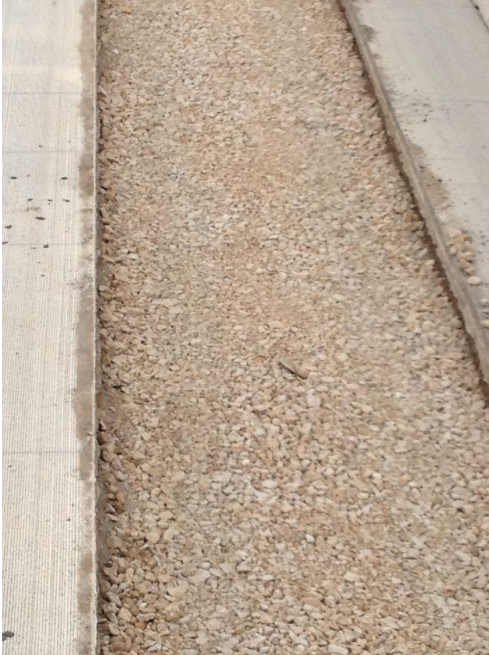
Figure C9. Base aggregate below concrete surface one-lane in width, consist of onsite RCA and RAP, imported RCA, and virgin aggregate (September 2015)
