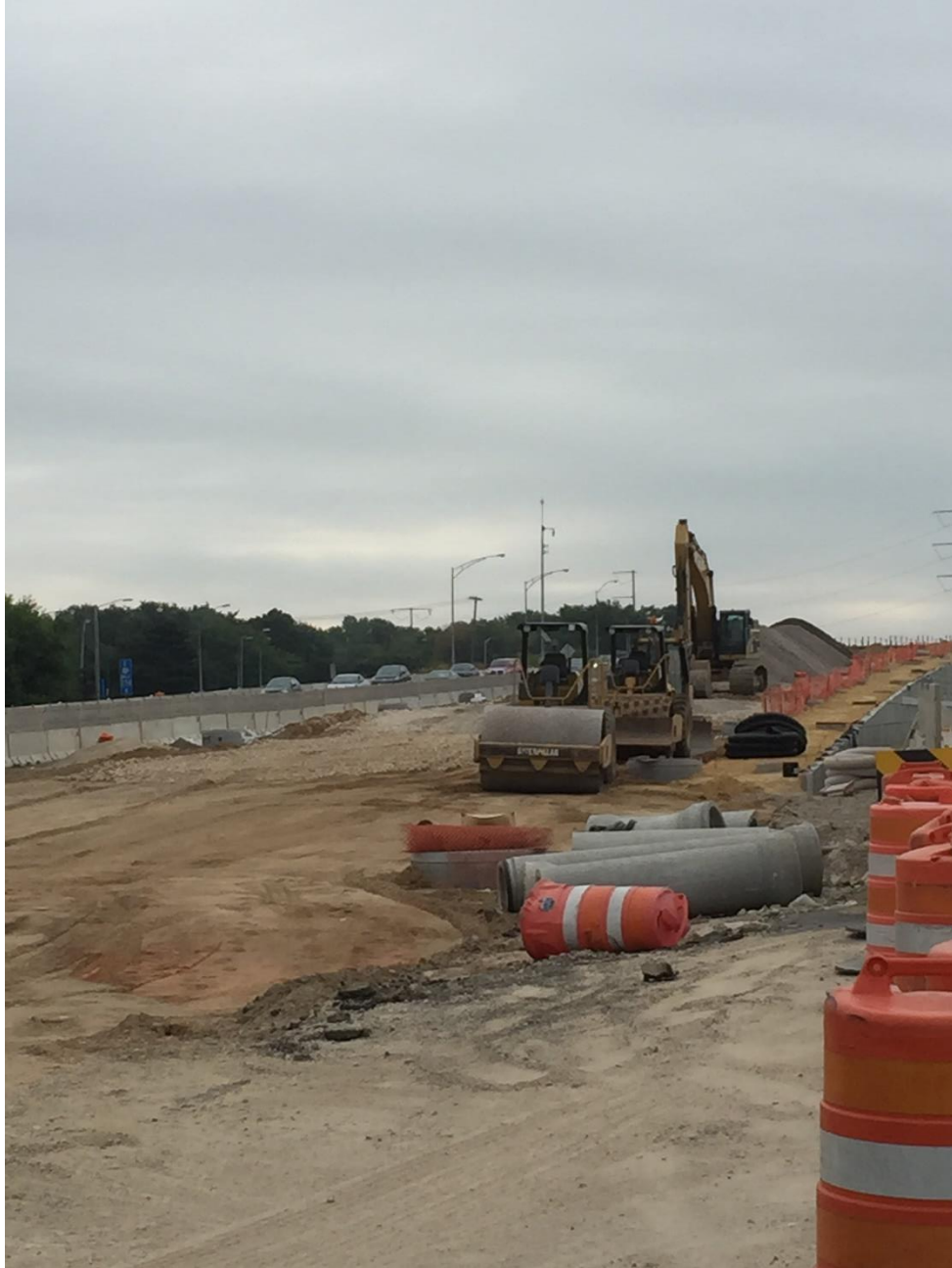
Figure C11. Construction of base course on one of project's bridges; aggregate is stockpiled in the background (September 2015)
