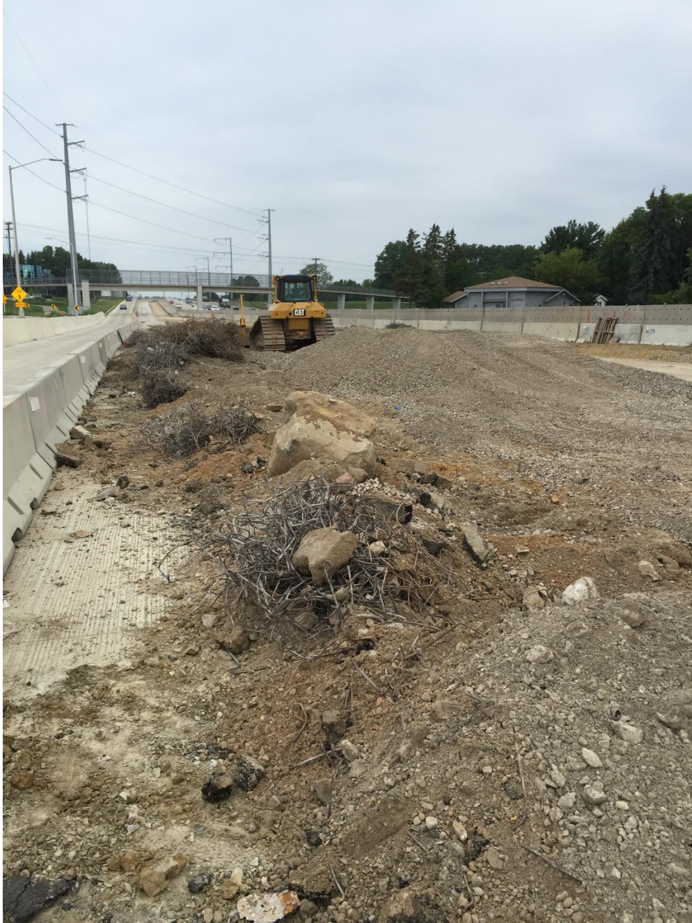
Figure C10. Onsite recycled pavement stockpiles; rebar is removed from existing pavement and discarded (September 2015)
