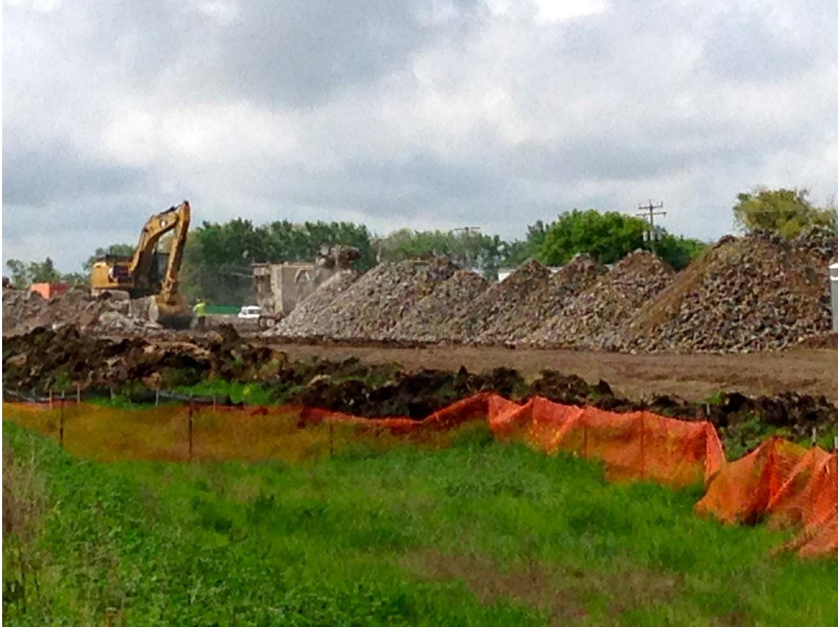
Figure C6. Photo of on-going concrete crushing for RCA; RCA stockpiled onsite (June 2013)
