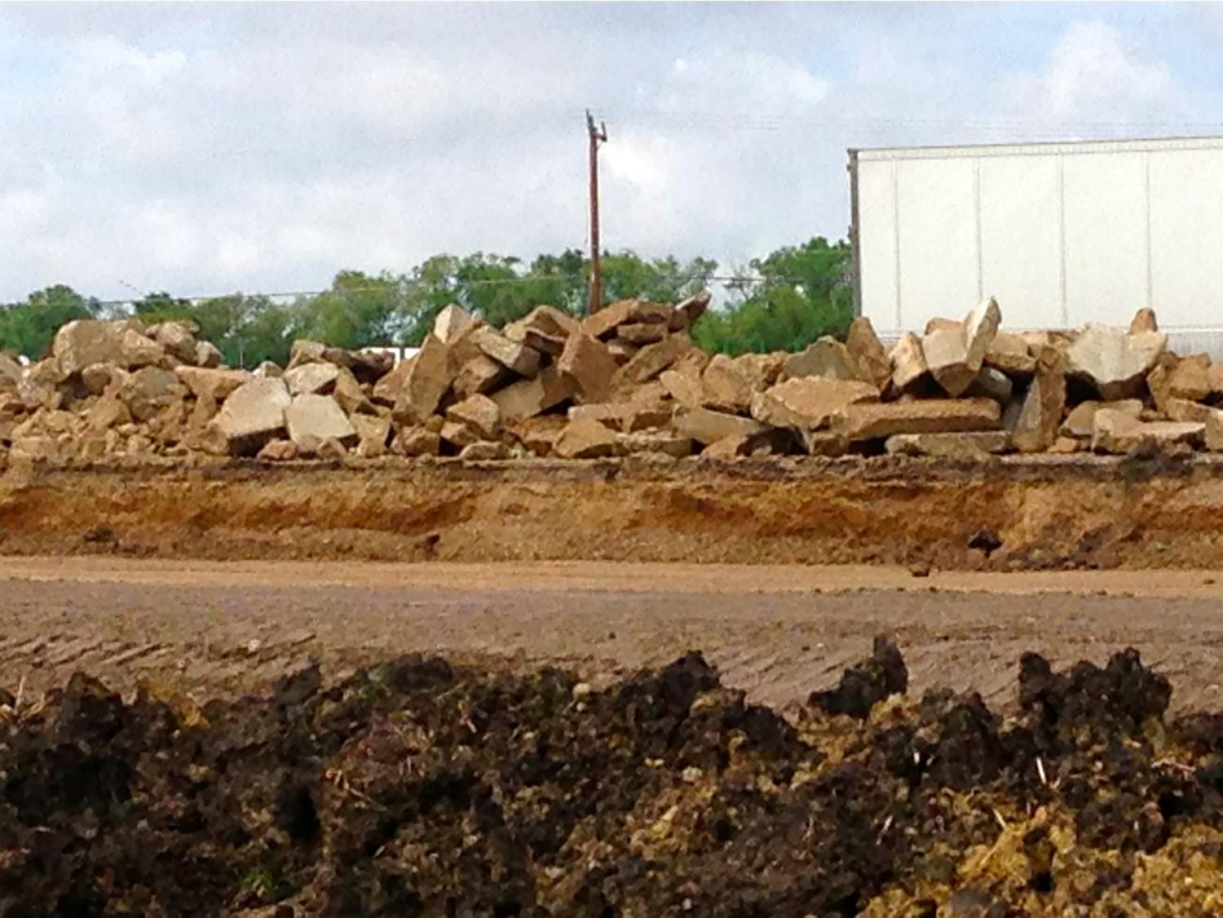
Figure C5. Demolished concrete pavement stockpiled onsite (June 2013)
