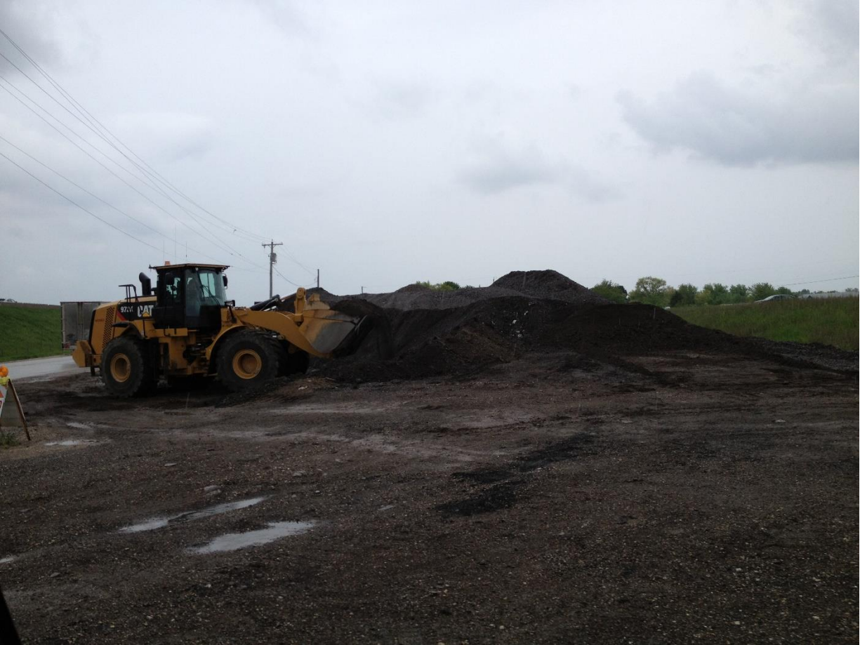
Figure C7. We Energies fly ash used in concrete mix; We Energies dug fly ash out from landfill nearby their coal power plant for use on the roadway (June 2013)
