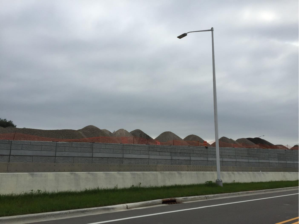
Figure C12. Recycled aggregate stockpiled onsite; space for stockpiling was sparse in urban environment and some piles were placed on bridge/ramp expansions (September 2015)
