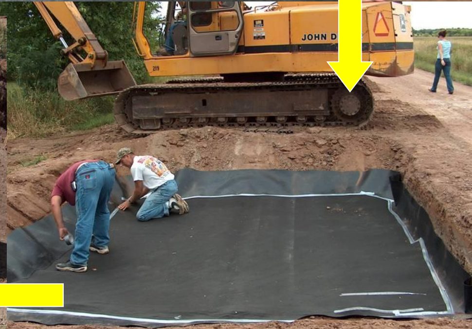
Drainage layer installation
