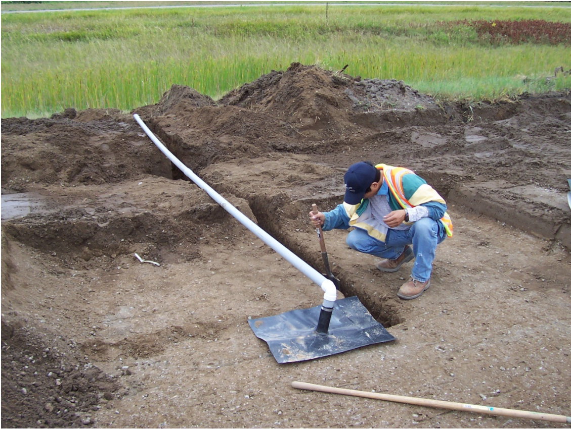
Figure A-2: Preparing drainage pipe from lysimeter to collection tank.
