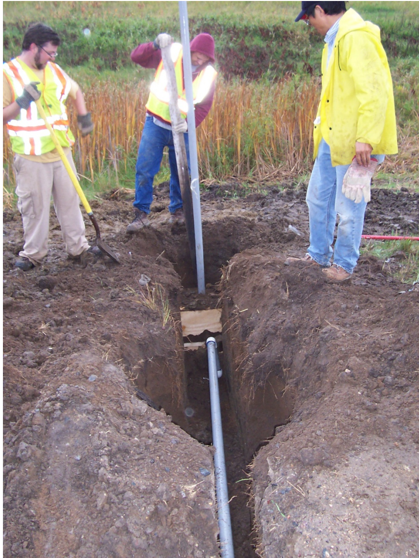
Figure A-8: Installing leachate collection tank.
