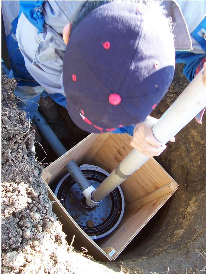
Figure A-7: Installing leachate collection tank.
