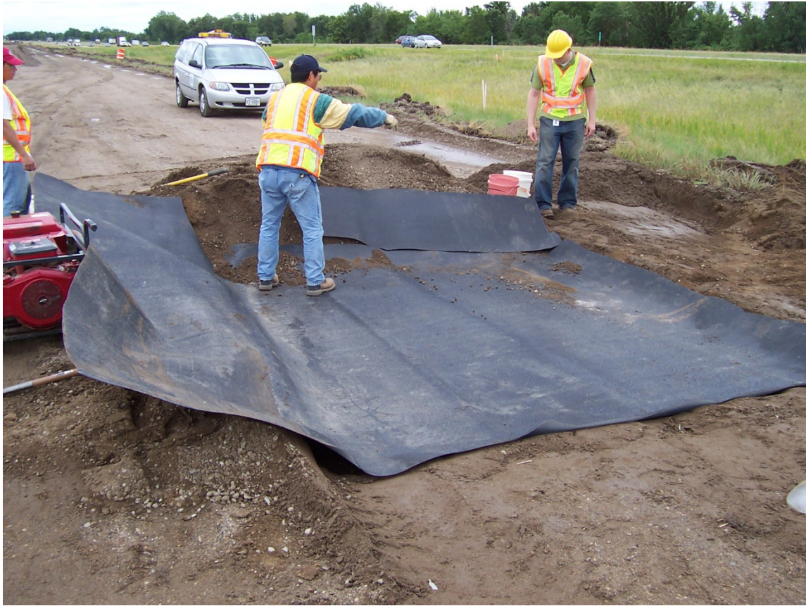
Figure A-3: Installing geomembrane for lysimeter.
