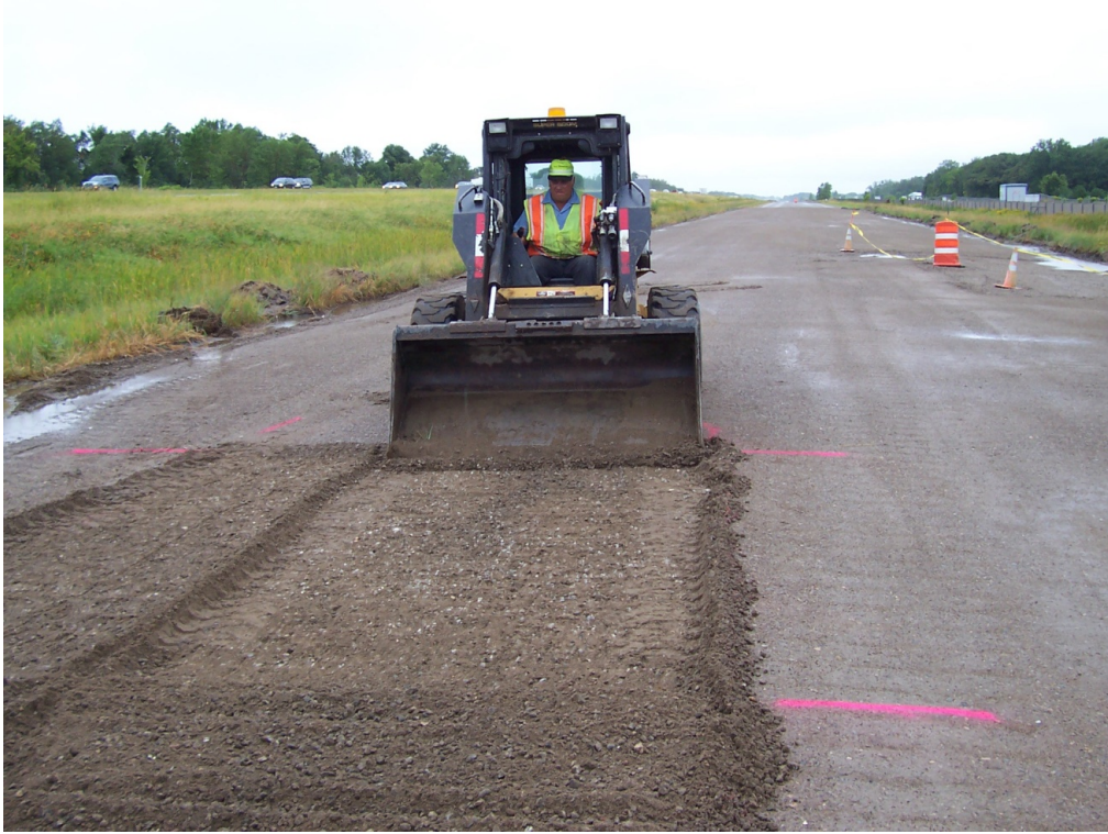
Figure A-1: Preparing indentation in sub-base for lysimeter geomembrane.
