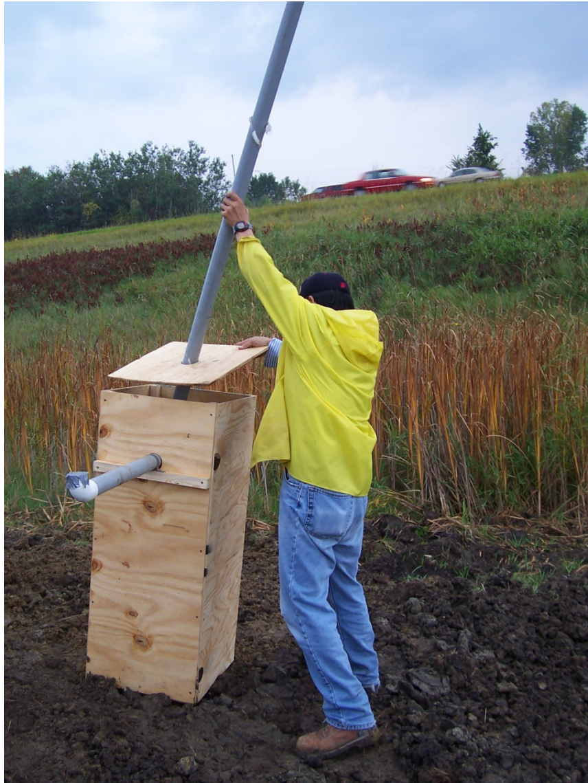
Figure A-6: Assembling leachate collection tank.
