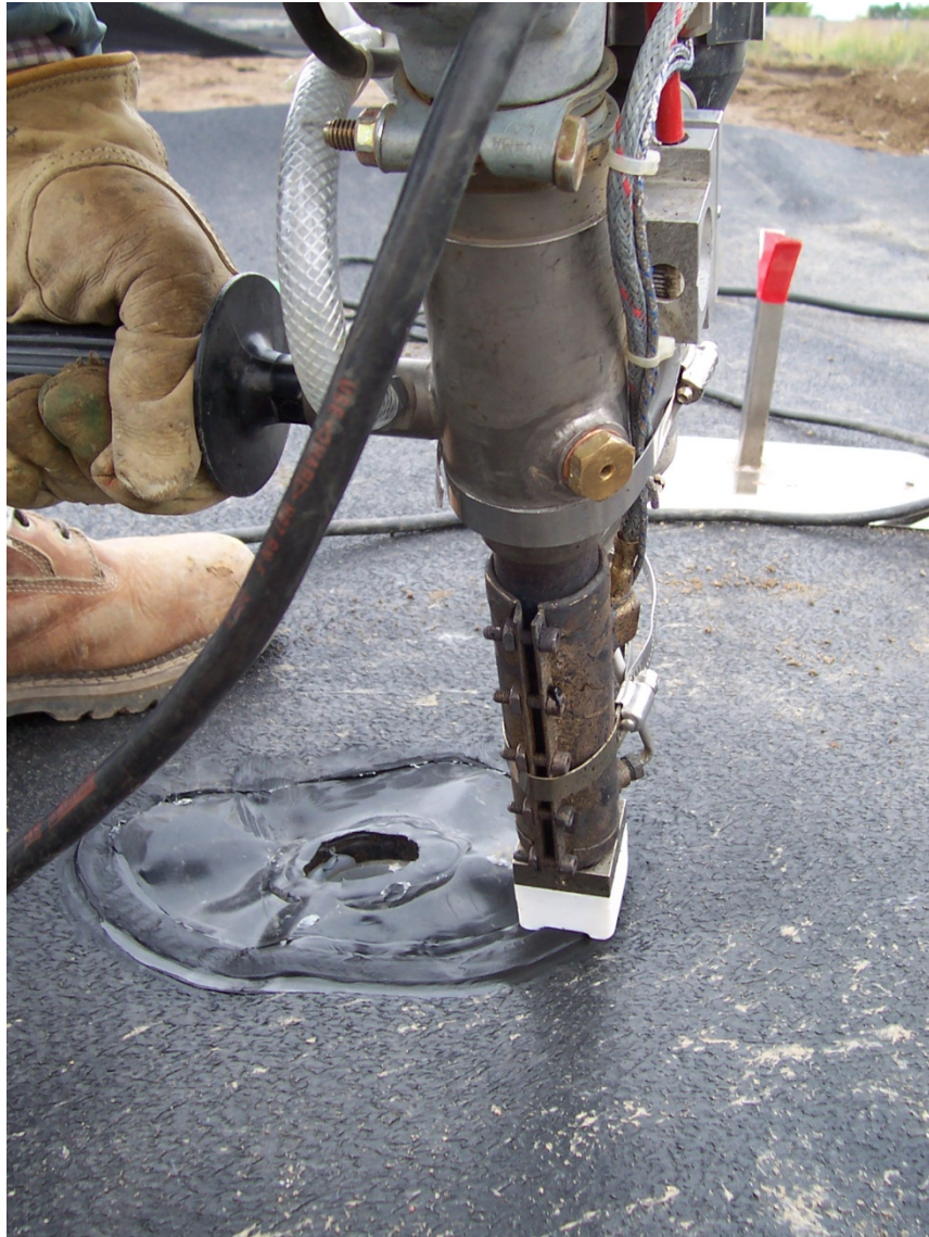
Figure A-4: Welding geomembrane to lysimeter drainage pipe assembly.
