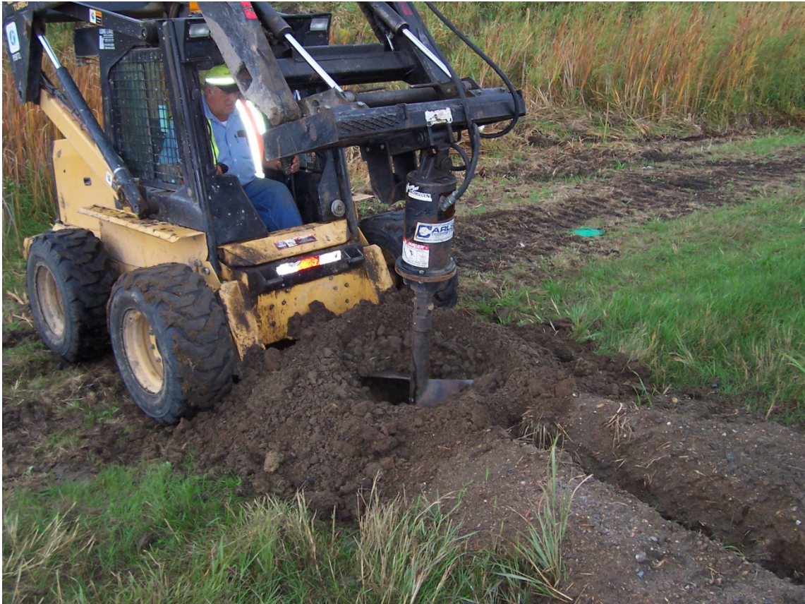
Figure A-5: Preparing hole for leachate collection tank and trench for drainage pipe.
