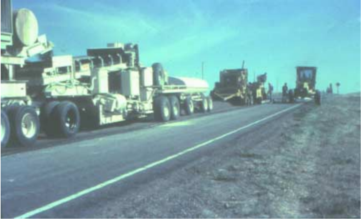
Figure 2. CIR Process, Site 1, US-283
