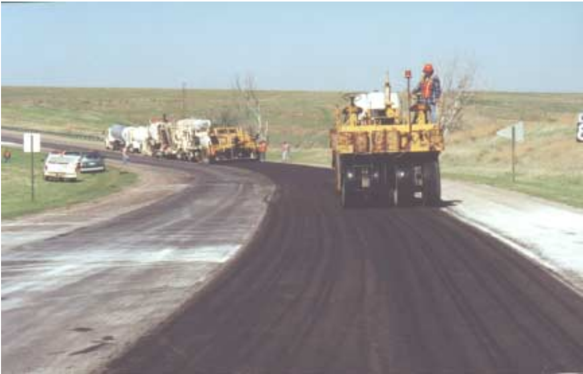
Figure 3. CIR Compaction, Site 2, US-24
