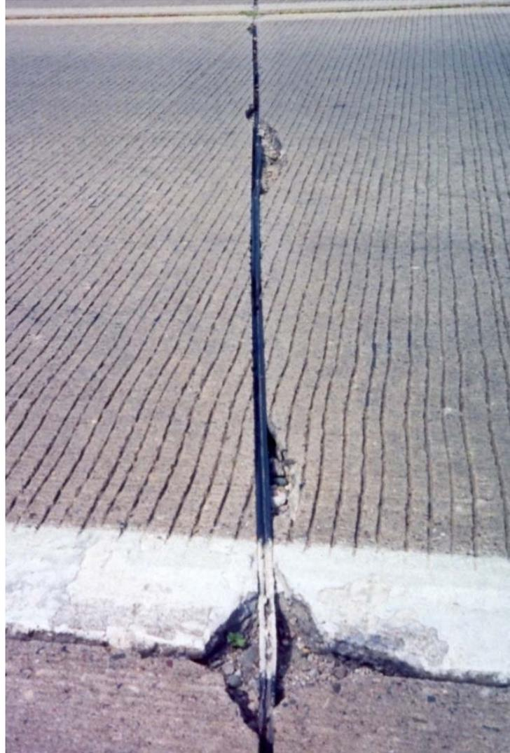
Figure 3: Severe Transverse Joint Spalling
