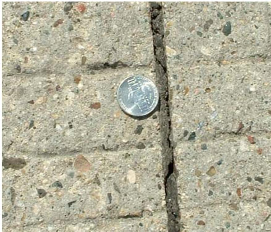
Figure 13: Typical Transverse Joint Width
