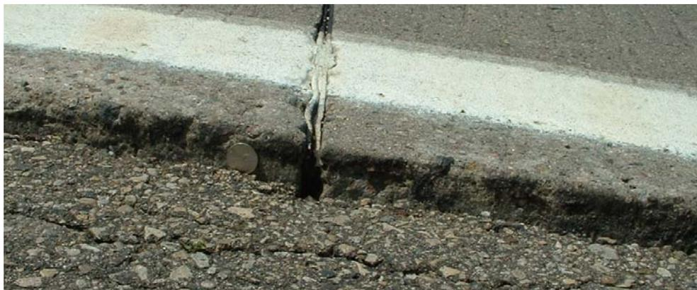
Figure 9: Severe Lane to Shoulder Drop off
