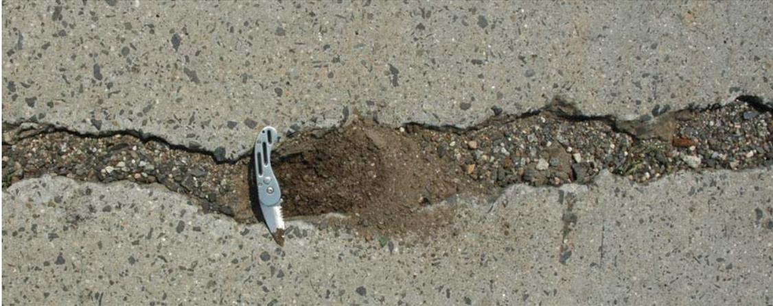
Figure 49: Typical Transverse Crack found on CT1-1 and CT1-2
