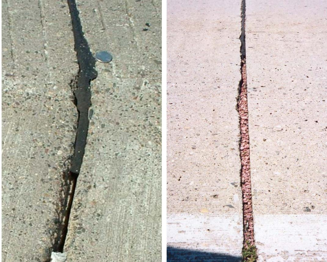
Figure 4: Transverse Joints with Seal Damage
