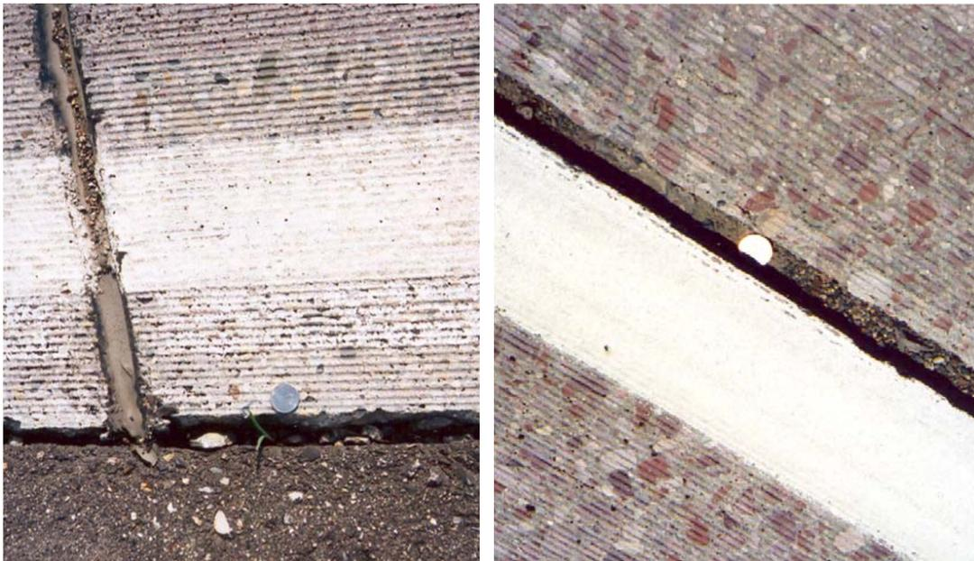
Figure 10: Typical Lane to Shoulder Separations
