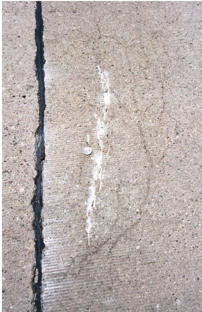
Figure 6: Severe D-Cracking at a Transverse Joint
