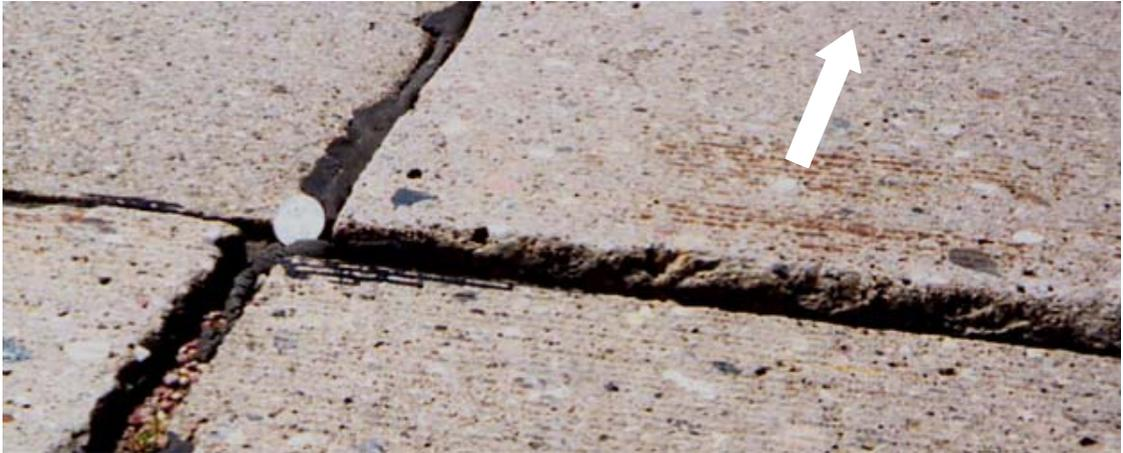
Figure 11: Large Faulting Between Panels
