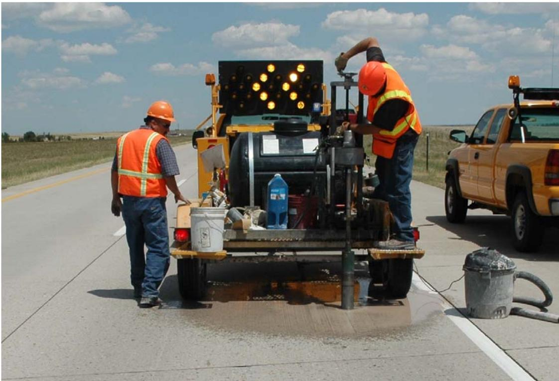
Figure 17: WYDOT Crew Members Extracting a Pavement Core
