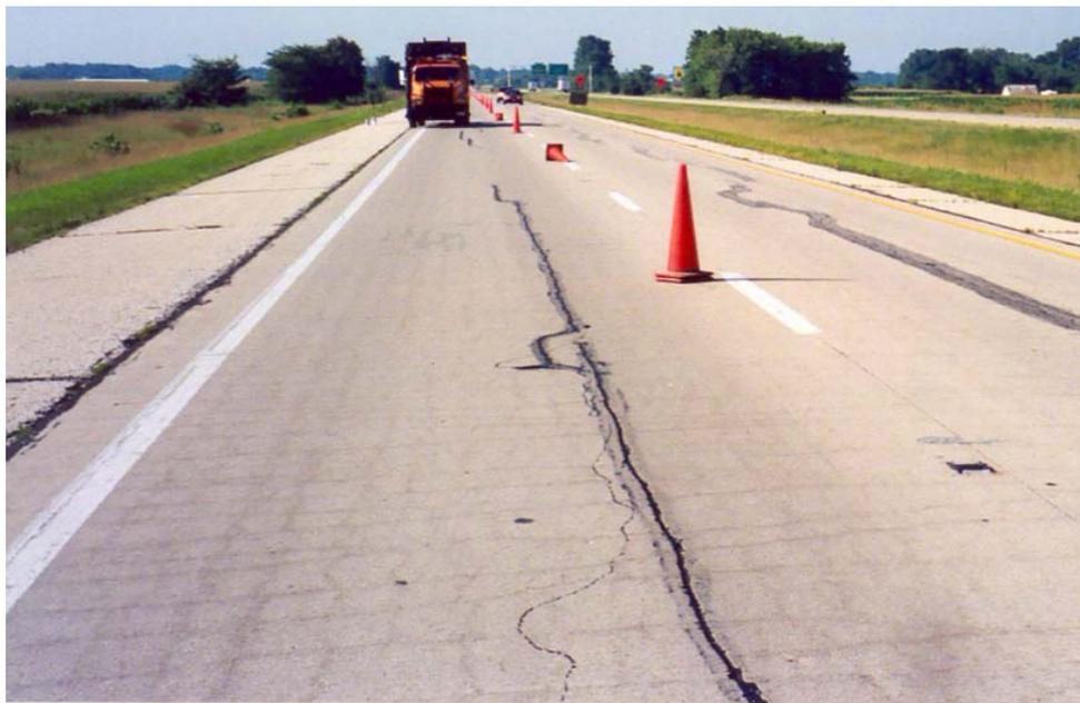
Figure 14: Medium Severity Longitudinal Crack
