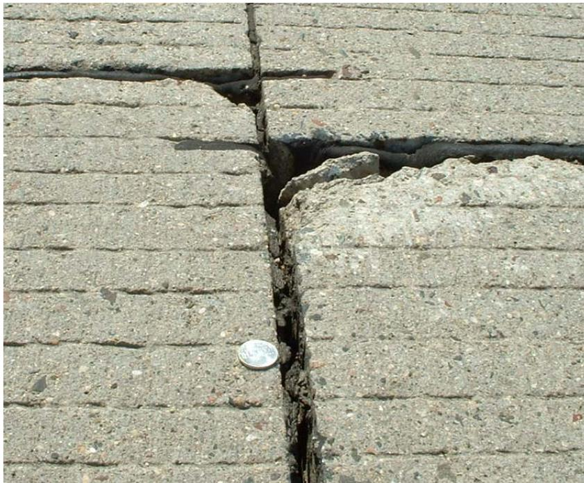
Figure 5: Longitudinal Joint with Seal Damage
