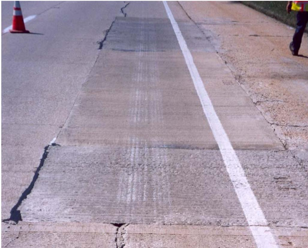
Figure 7: Slab Patch Intersection with Distress
