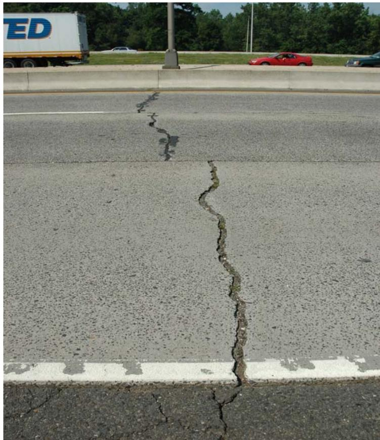
Figure 15: High Severity Transverse Cracks
