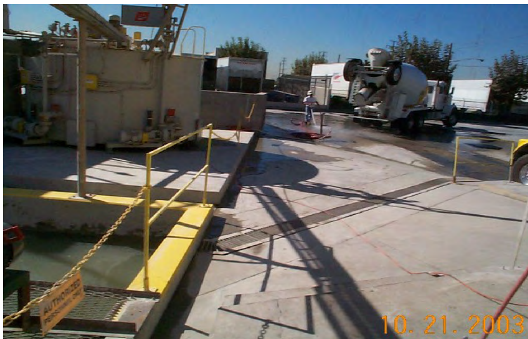
Figure 28. Washout Water Drain System. Red-I-Mix Concrete Inc. Facility Visit. Irwindale, CA.
