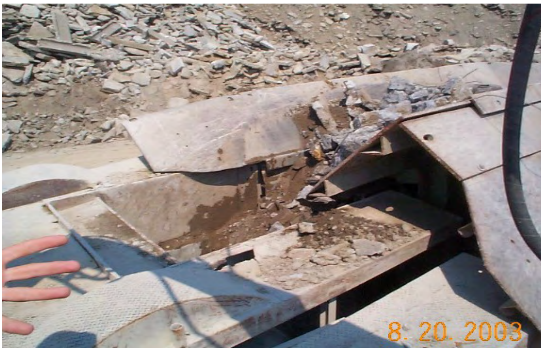
Figure 8. Primary Crusher. . Iafrate Crushing Plant Visit. Taylor, MI
