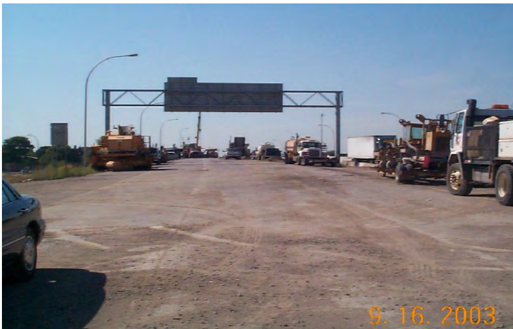
Figure 16 I-694 Reconstruction Project Visit. Brooklyn Center, MN.
