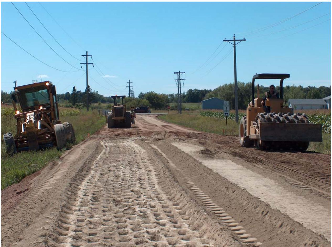
Fig A9. Compaction of fly ash and RSG mix by using sheep foot and roller drum compactors.
