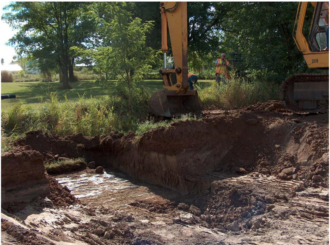
Fig A14. Excavation of lysimeter pit.
