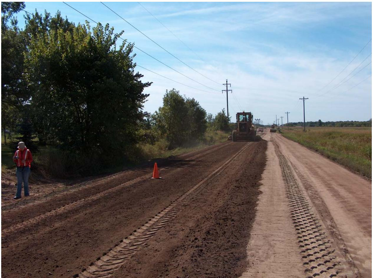
. Fig A10. Compaction and grading of S-RSG surface.
