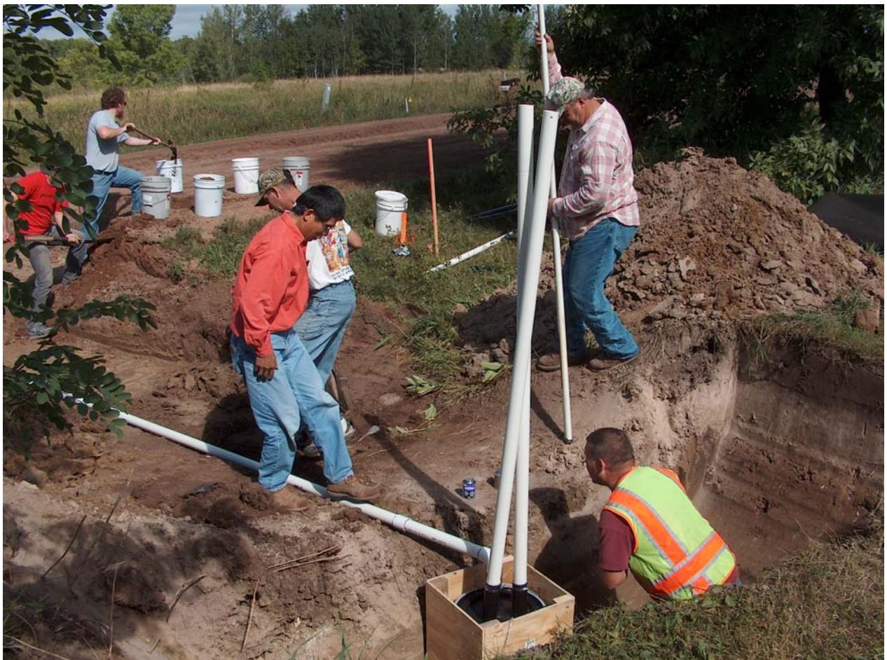
Fig A15. Construction of water tank and lysimeter – tank connection pipe.
