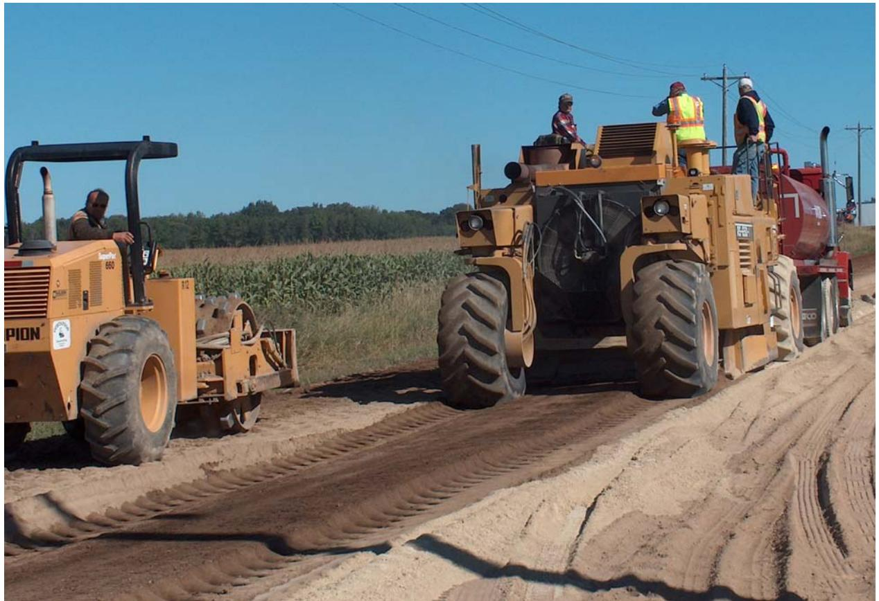
Fig A7. Road-reclaimer blending fly ash and water truck
