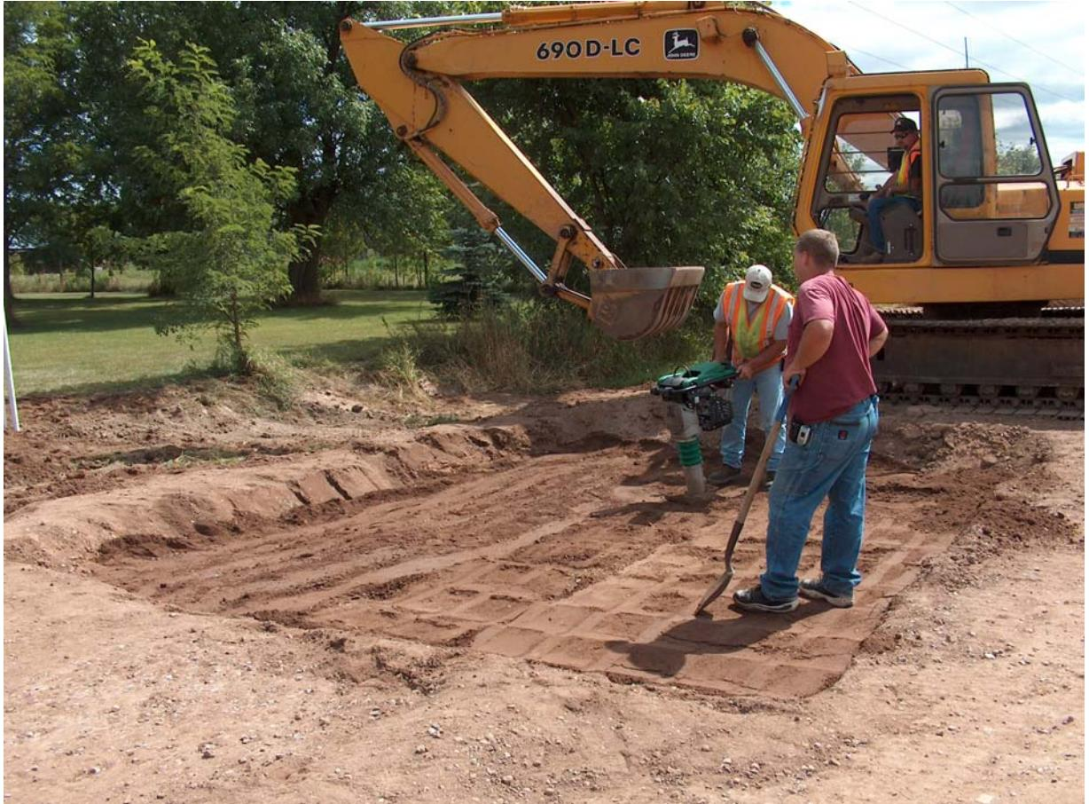
Fig A17. Controlled filling of lysimeter pit with subgrade and RSG.
