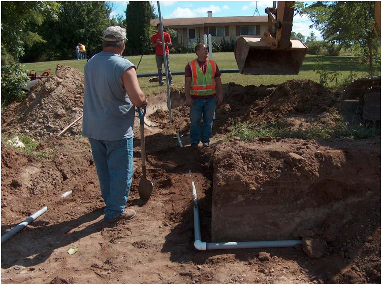
Fig A19. Installation of temperature sensors into subgrade and RSG in lysimeter pit.
