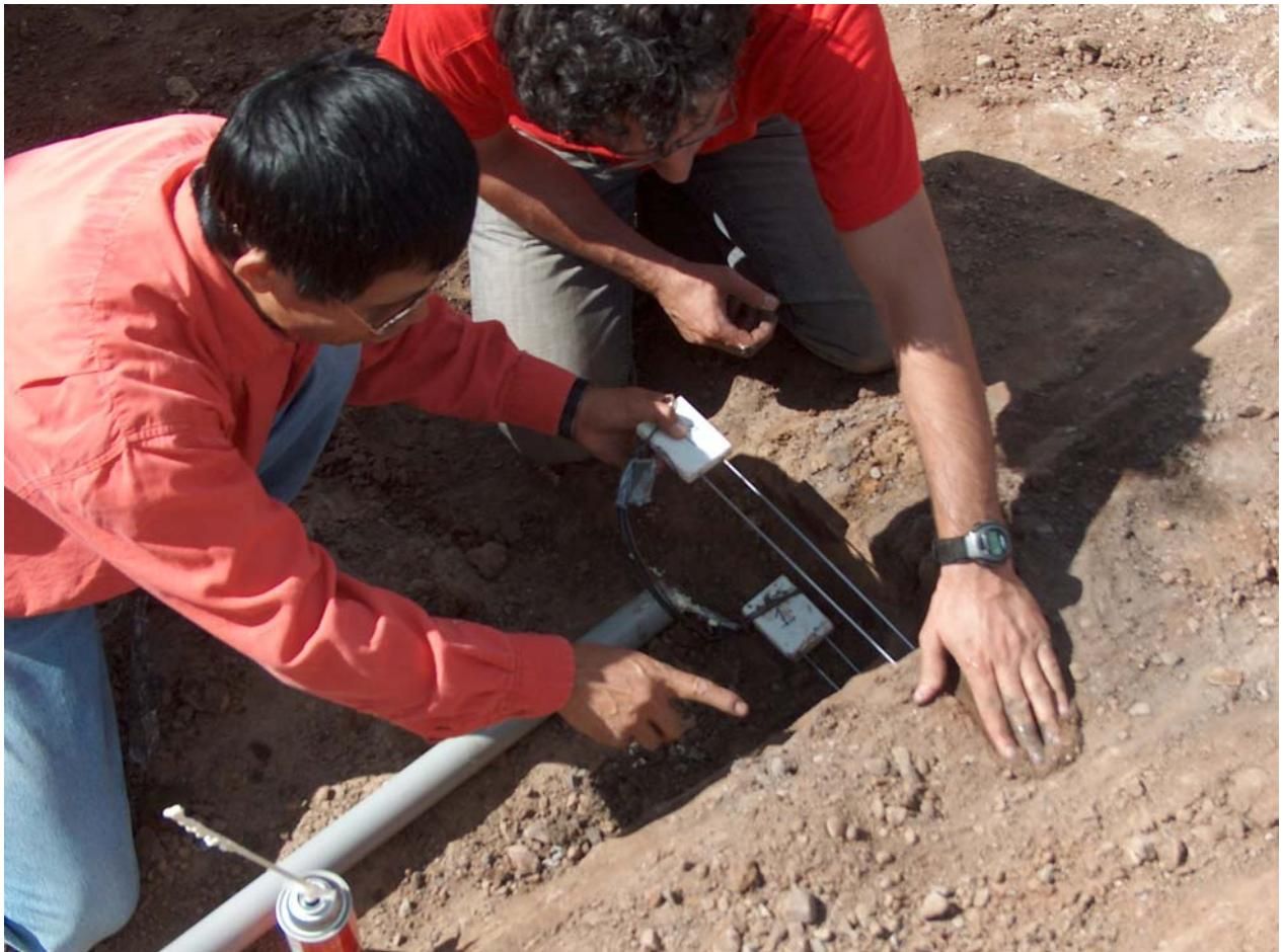
Fig A18. Installation of volumetric water content and temperature sensors into subgrade and RSG in lysimeter pit Sensor 1 is in subgrade and Sensor 2 is in RSG.
