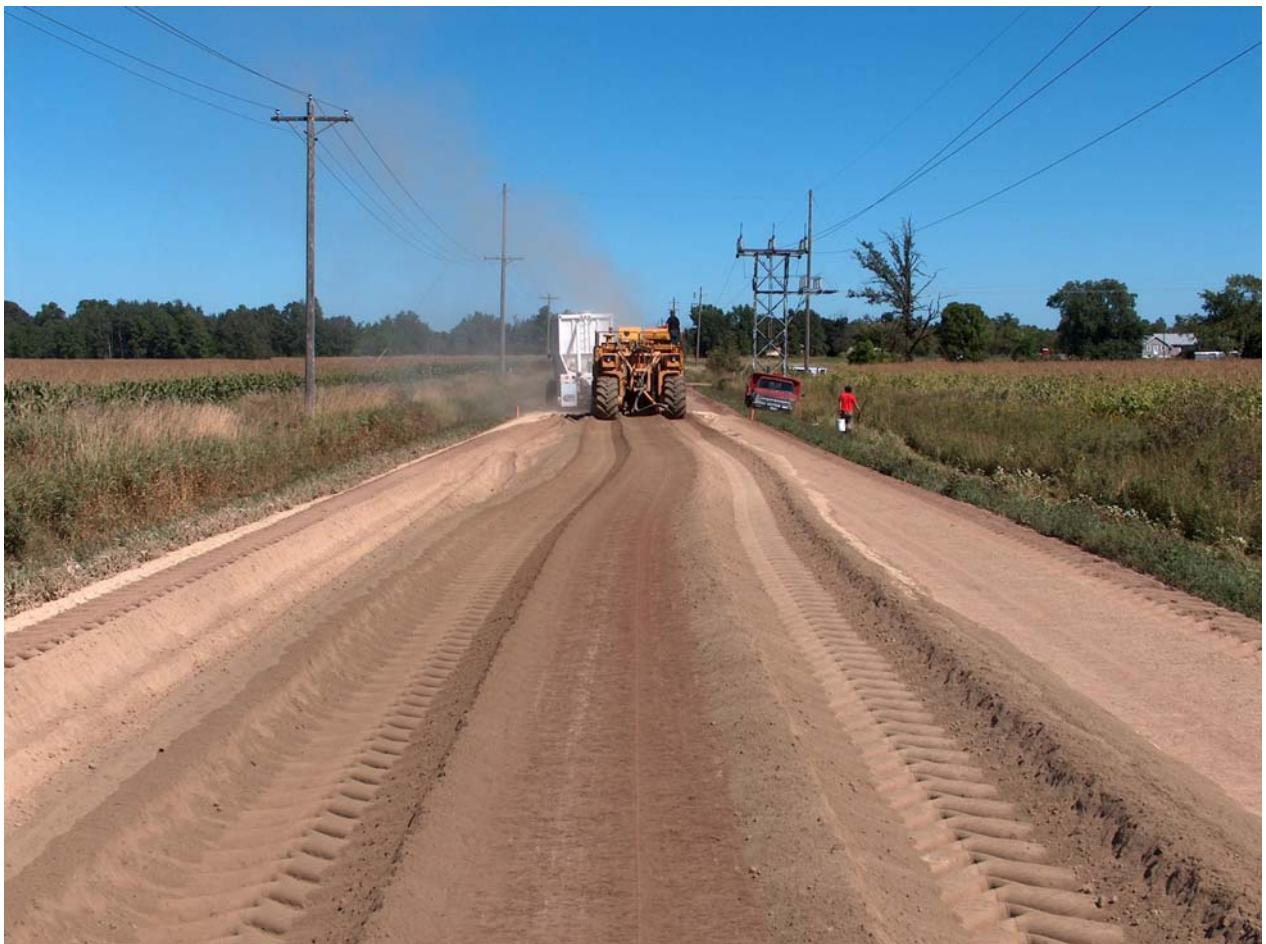
Fig A8. Road surface after blending process.
