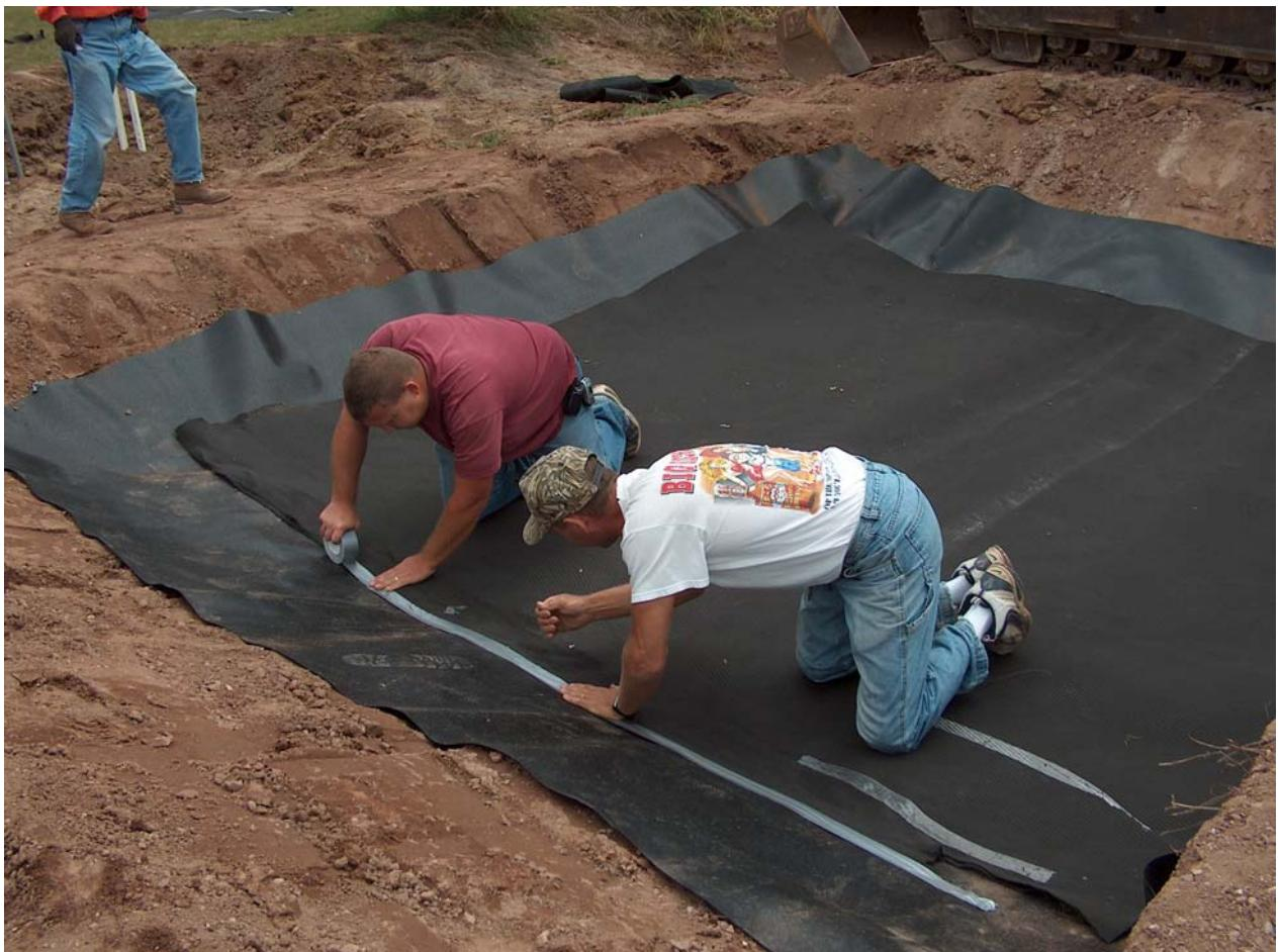
Fig A16. Placement of geomembrane and geotextile.
