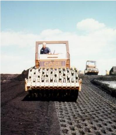
Foundry sand being compacted at STH 60
