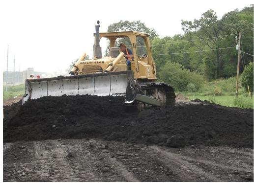
Foundry sand being spread as sub-base at STH 60 field site.
