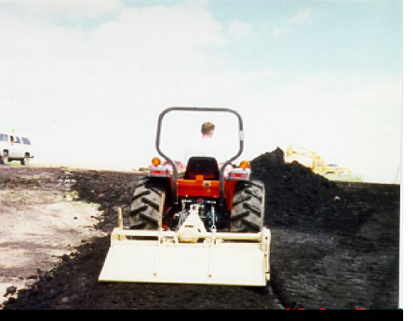
Disking or rototilling sand improves moisture distribution significantly, but is only required if strict control on water content is required.
