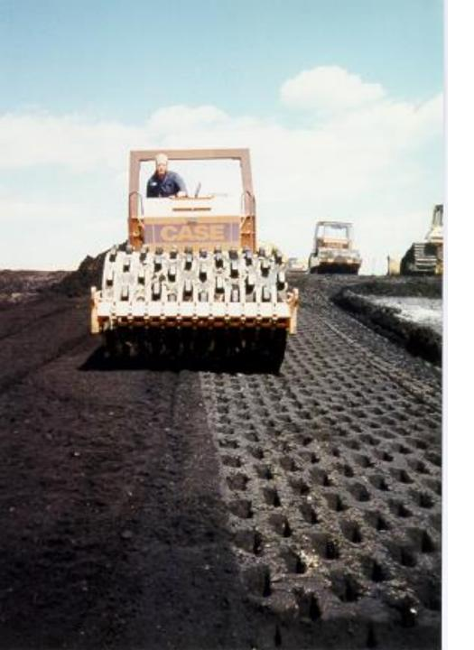
Compacting green sand with a footed roller improves compaction. Padfoot compactors work best.
