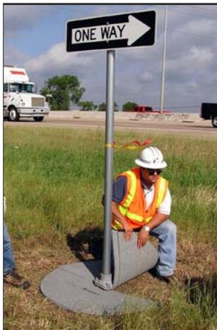
evaluate the ease of installation, cost, and effectiveness of anti-vegetation tiles made from recycled tires. The tiles are designed to control vegetation around guardrails and signposts. Nine TxDOT district offices in various parts of the state are taking part in this demonstration project, including: Austin, Beaumont, Childress, Corpus Christi, Dallas, El Paso, Lufkin, Pharr, and
