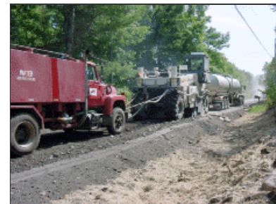
Reclaimer pushing the asphalt tanker and introducing the foamed asphalt into the base.
