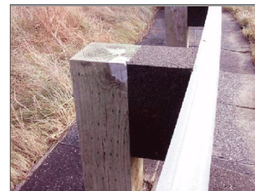
Spacer block manufactured from recycled tires.
