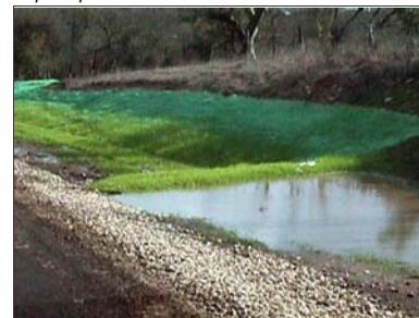
Follow-up photo of slope that was protected using a compost blanket. The slope shows thick, uniform vegetation and no evidence of erosion.
